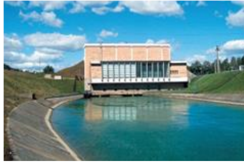
Fig. 1. Cerbureni power house – downstream view.
