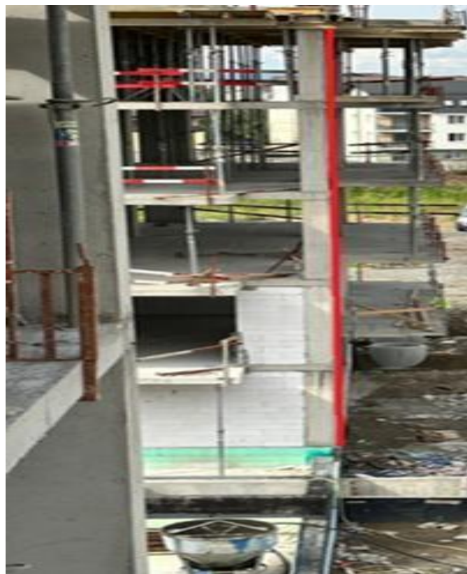
Fig. 5. Checking the verticality of the structure
