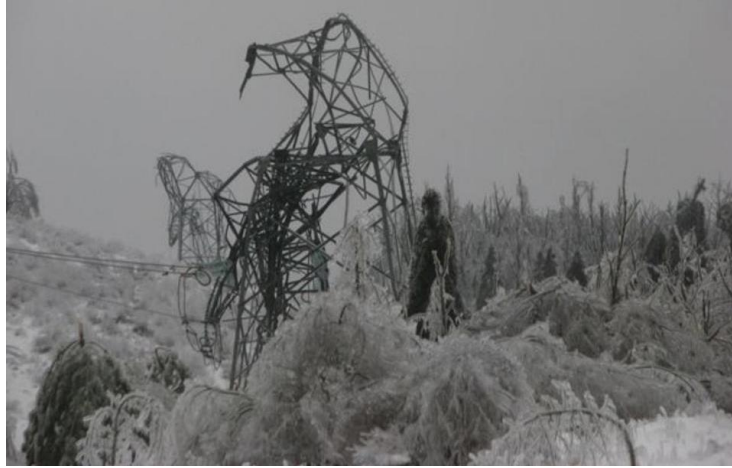
Fig. 6. Icing of an overhead line.
