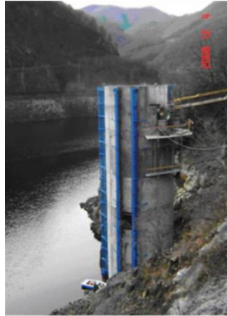
Fig. 5. The new intake tower.
