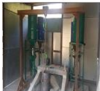
Fig. 17. Equipment placement in the aluminothermic steel mill demonstrator.
