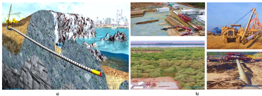
Fig. 2. Installation of fluid transport pipe by HDD method (overview).
