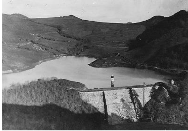
Fig. 3. Taul Mare Dam general downstream view (1936 photo).
