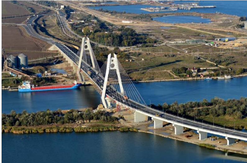
Fig. 12. Airy view of cable-stayed bridge over Danube - Black Sea Canal at Agigea
