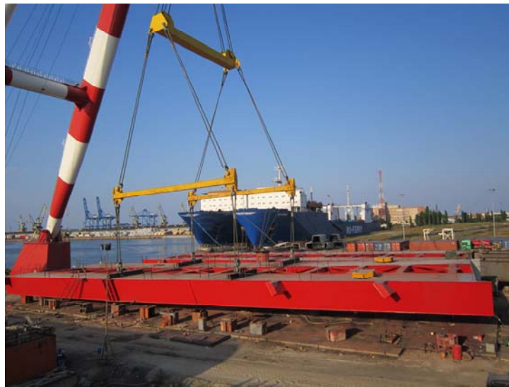
Fig. 7. The two segments of the steel deck over the pylons
