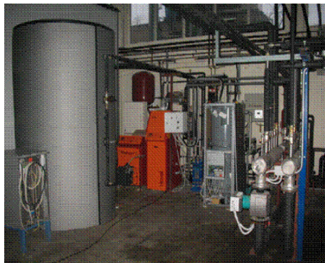
Fig. 7. YAZAKY type absorption refrigerating system with lithium bromide-water solution
