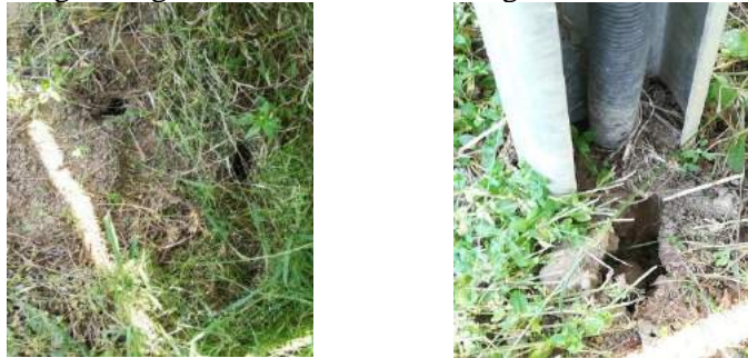
Fig. 15. Rodent traces found near the cable routes between the strings of PV panels.
