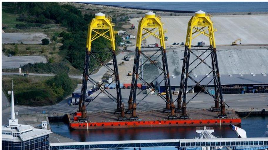
Fig. 8. Jacket foundation for the Wikinger offshore wind farm [12]
