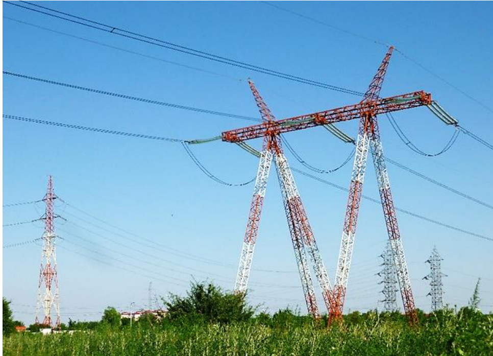
Fig. 2. The high voltage overhead 400 kV' power lines for which magnetic field measurements were performed.
