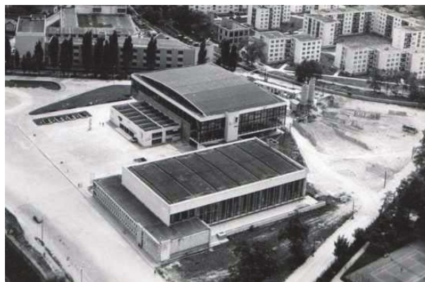
Fig. 4. The top view of the new building - Sports Hall officially opened in 1965 – rear end [8].
