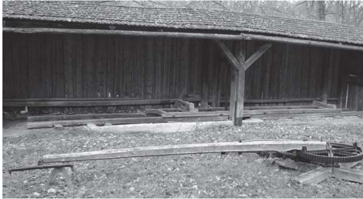
Fig. 1. The shed where the saw mill it is assembled.
