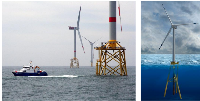
Fig. 9.a) Jacket foundation in foreground and monopile structure in background, at Alpha Ventus [14]; b) Twisted jacket foundation [14]
