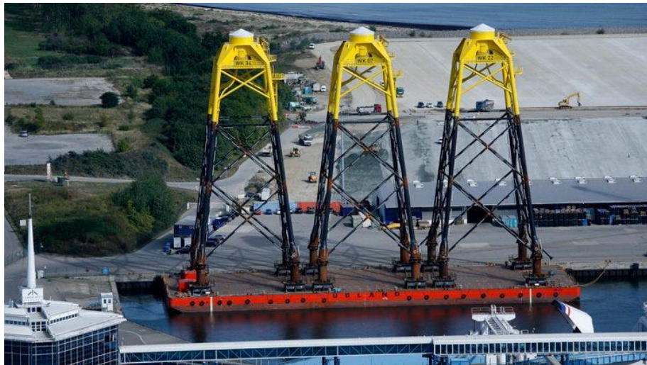
Fig. 8. Jacket foundation for the Wikinger offshore wind farm [12]
