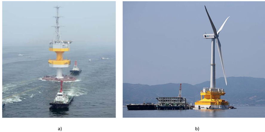
Fig. 16. a) Towing of converter platform; b) Fukushima Hamakaze turbine being towed to final location [27]
