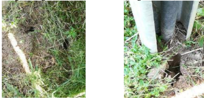
Fig. 15. Rodent traces found near the cable routes between the strings of PV panels.
