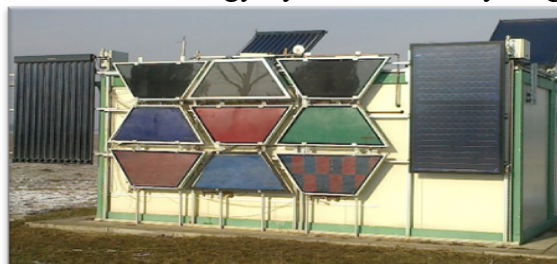
Fig. 2. Solar-thermal array with trapeze flat plate solar-thermal collectors for architectural integration.
